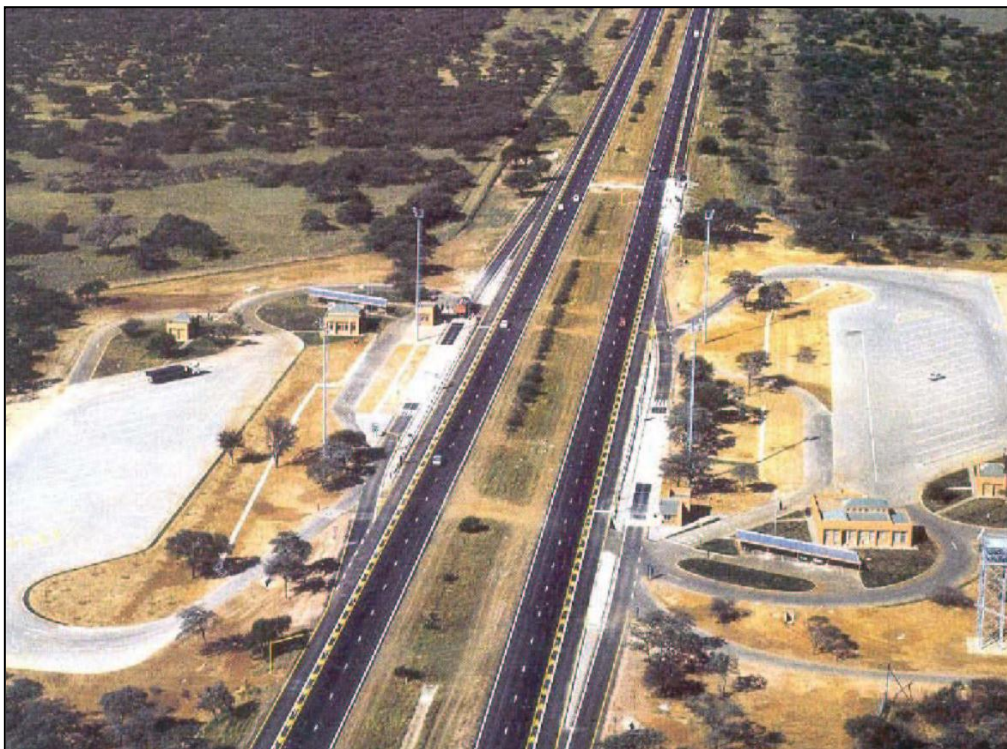
Aerial view of Mantsole weighbridge facility on N1
