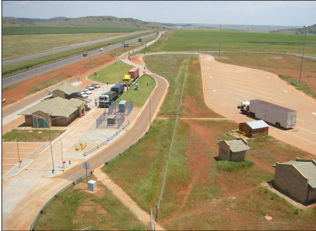
Aerial view of Heidelberg West weighbridge facility on N3
